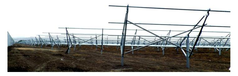
The assembly method, with driven piles, mounting rails and components, is very flexible and gives to the constructors the ability to work fast and to encounter any problem or obstacle.
