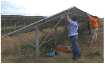
The structue is well balanced, so a small crew of 4-5 persons can easily adjust the inclination of every stand.
